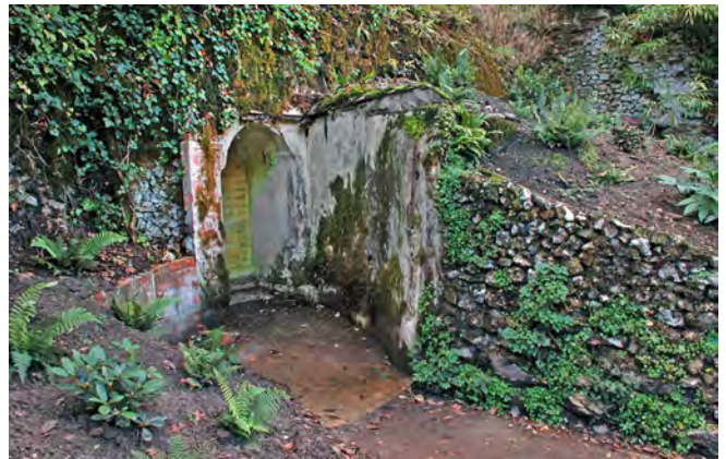
Two of the three entrances to the WWII bunker
